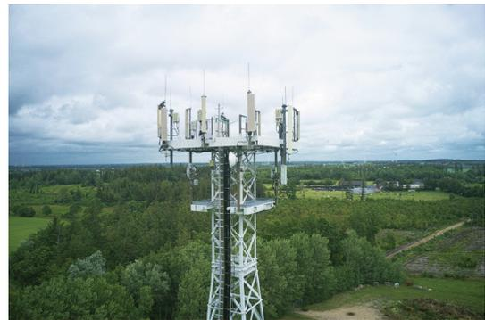
**Fig. 1.** 5G towers like this one are now transmitting at frequencies that are close to the frequencies used by aircraft altimeters. Expanding service to these frequencies offers better performance for cell phone users but could interfere with the proper functioning of some altimeters. Credit: Fabian Horst (CC BY-SA 4.0).
